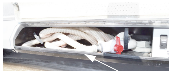
Sewage Drain Hose (Located in water service center) -Typical View
